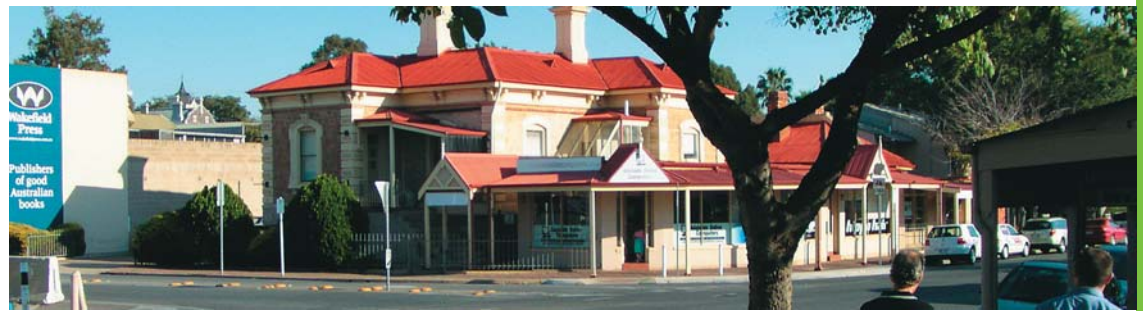
Our new premises at 58 Rundle Street, Kent Town
